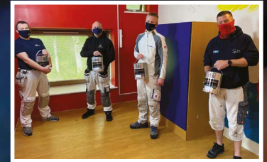
Revamping the bedrooms at Treetops
